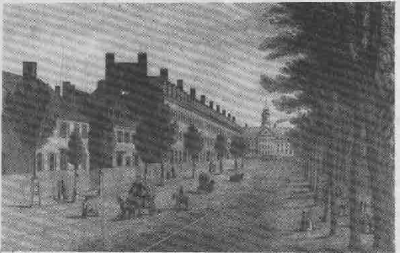
A view of Dutton Street, Lowell, Massachusetts, in the 1830's showing the mills and boarding houses of the Merrimack Manufacturing Company, where some of our Rice cousins worked and lived. These buildings were all razed in 1960.
